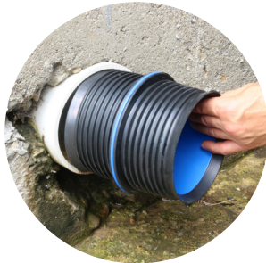
2) Lubricate gasket O.D. with soap & water solution
