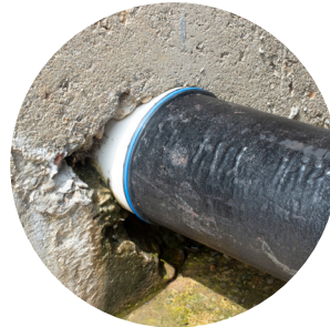
4) Lubricate gasket and install 2nd pipe
