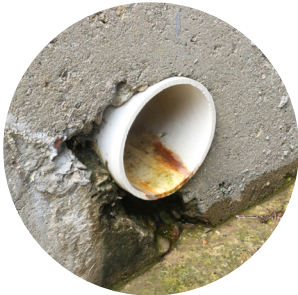
1) Clean and measure pipe I.D.
